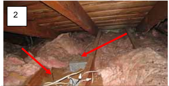
Item 26 - Bathroom ceiling exhaust fan vents into the attic and there is an absence of insulation.
