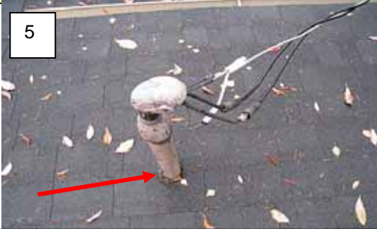
Item 1 - No flashing what so ever around the electrical service mast.
