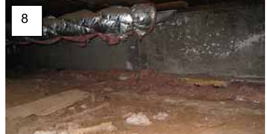
Item 32 - Lots of debris and missing vapor barrier.
