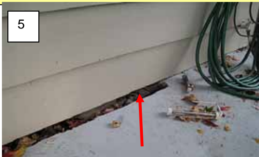
Item 5 - Unscreened opening to under the family room area.
