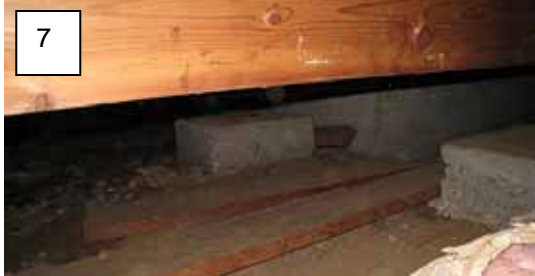
Item 32 - Lots of wood debris on the ground in the crawlspace.
