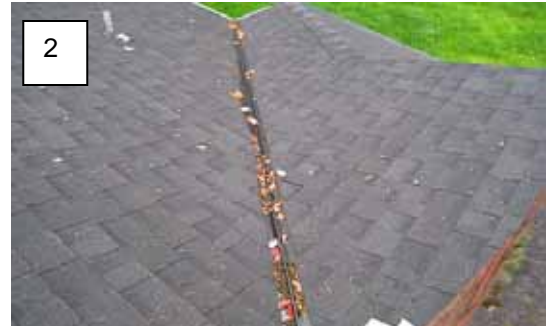
Item 1 - Shingles along the valley are sloppily cut.
