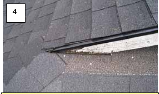
Item 1 - The roofing is installed wrong at the north end of the end rafter on the west
