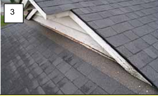
Item 1 - Roofing installation is incomplete at the west gable. Bare decking is
