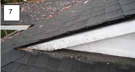
Item 1 - East gable has no flashing.
