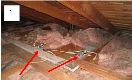
Item 17 - Open junction boxes with splices hanging out over the bathroom.
