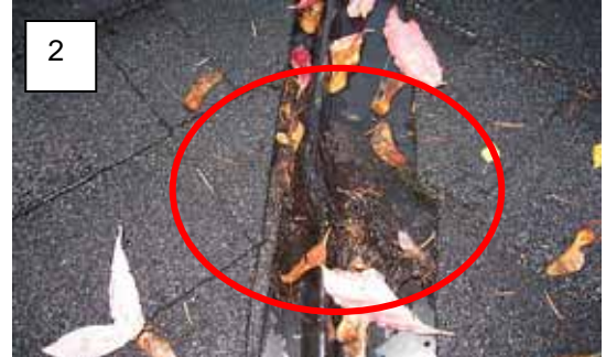
Item 1 - Sloppy valley installation, misaligned valley metal all gooped up with copious amounts of black sealant.
