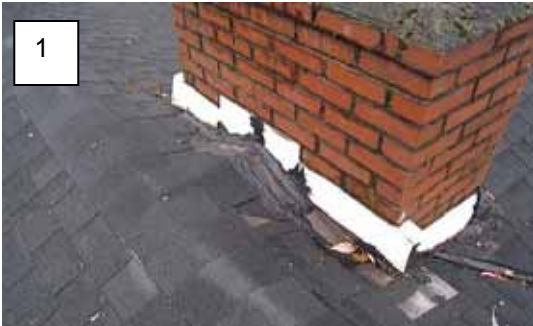
Item 1 - Another view of improperly flashed in chimney.
