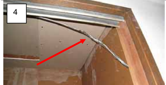
Item 18 - Unprotected and improperly installed NM cable runs in the furnace water heater closet.
