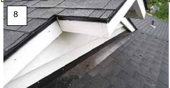
Item 1 - North gable has the sidewall flashing not counter flashed.
