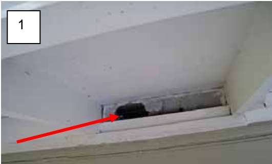
Item 4 - Torn open eave vent screen on the back of the house next to patio.
