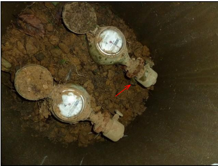
#1 meter well - pipe connect under here
