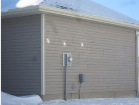
This view shows the effects of the thermal distortion on the siding on the north side of the garage.
