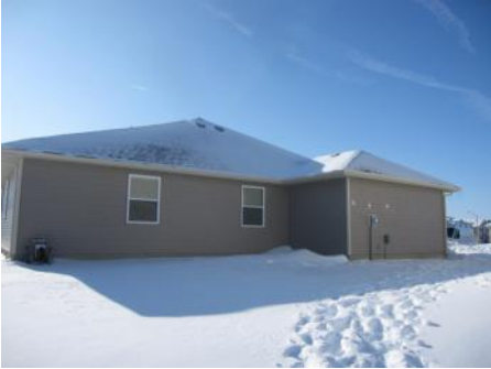
This view shows the effects of the thermal distortion on the siding on the north side of the garage.
