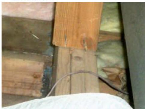
*The ceiling joists are not secured and are pulling away from the headers. Have a qualified contractor further evaluate and repair to reduce the risk of continued deterioration.*
