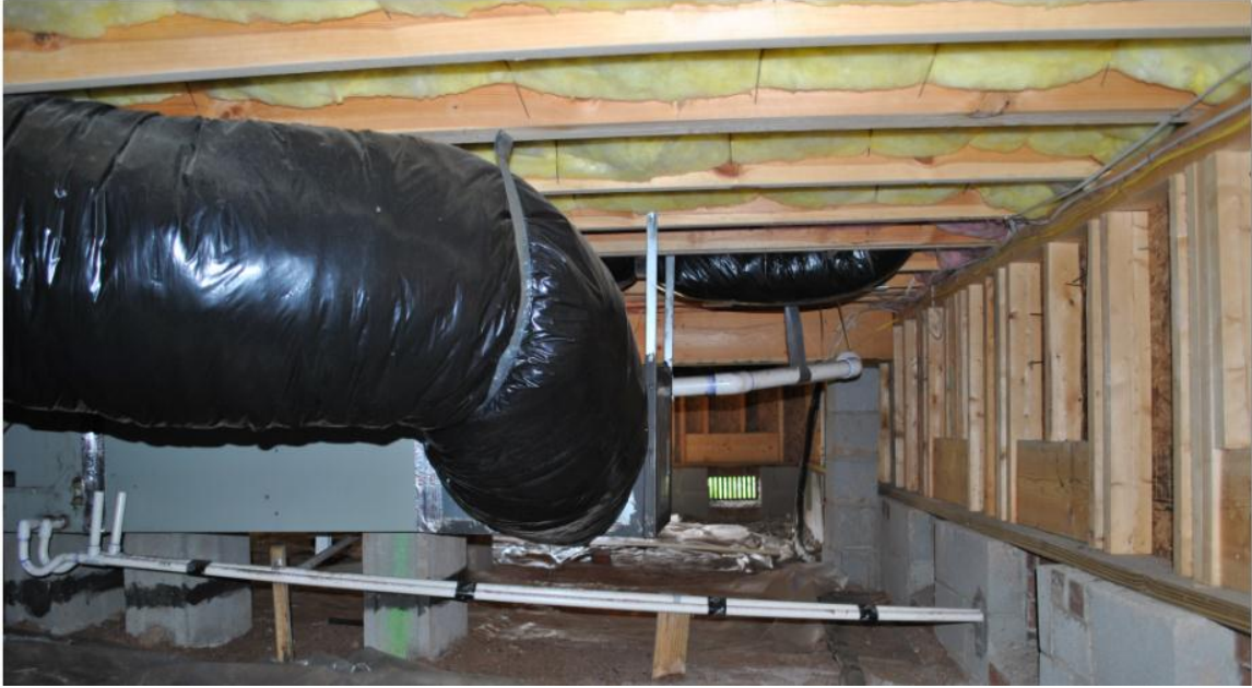
This one shows the entrance of the crawlspace.
